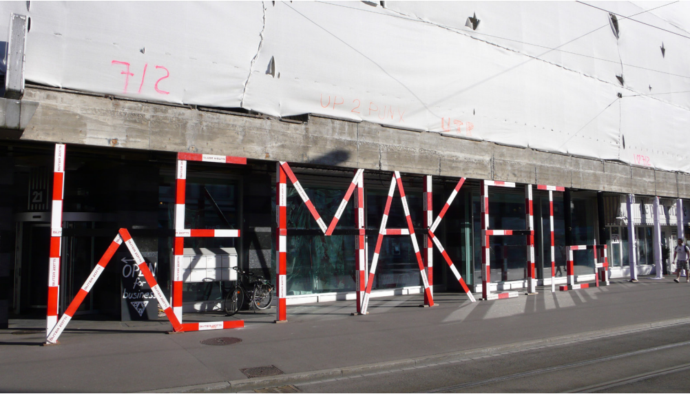
Construction site aesthetic: scaffolding with wemakeit.ch, Zurich 2012 (Photo: Private Archive of Michael Surber [p])
