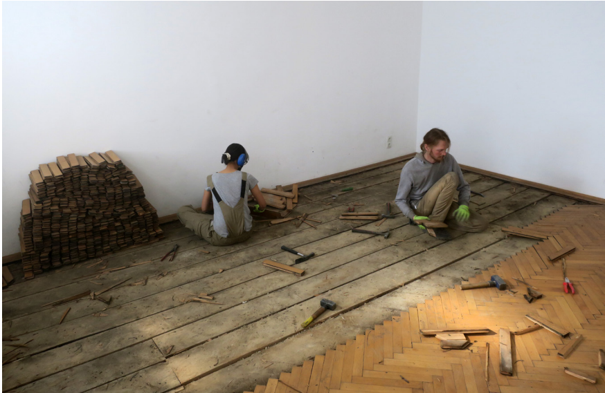
Manual salvaging of individual parquet slats from a Gründerzeithaus (tenement housing from the 19th century) in Vienna's inner-city district. The slats will be refurbished by the industrial producer before being reintegrated into new buildings. (photo: Madlen Kobi, 2022)
