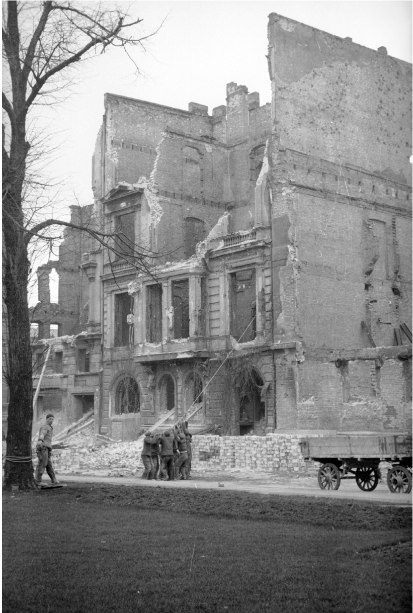
Demolition of a building damaged during the war in Wrocław, 1949. The workers are using the ›rope method‹ (pulling the wall down with a metal rope), which was the most popular way of demolishing ruins in postwar Poland.
